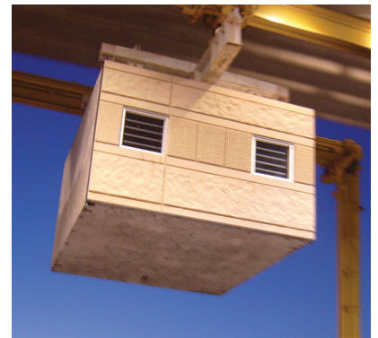
The prison modules were stacked into three towers surrounding a central courtyard, creating seven-story buildings. Photo: Tindall Corp.
