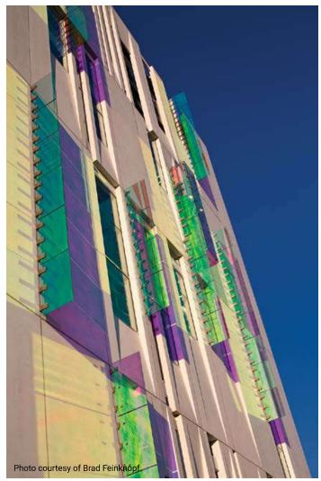
The dichroic glass fins reflect varying colors onto the precast concrete panels based on the angle of the sun.
